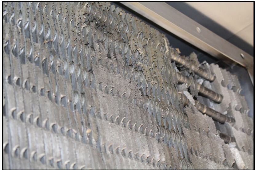
Aluminum fins severely corroded by application of highly alkaline (pH > 9.0) cleaning chemicals.
