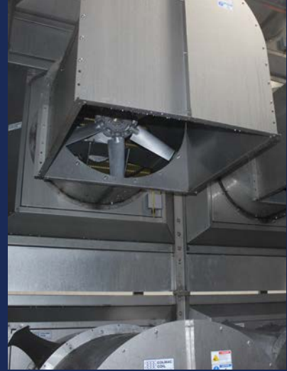
Defrost Hoods that trap defrost heat to shorten defrost cycle
